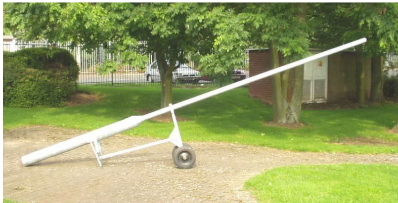
Figure 10-1 - Column installed on the carrier
