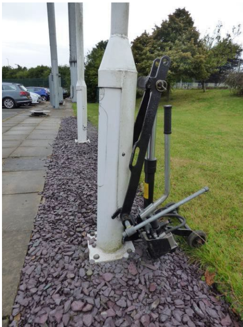
1. Attach counterbalance to column
