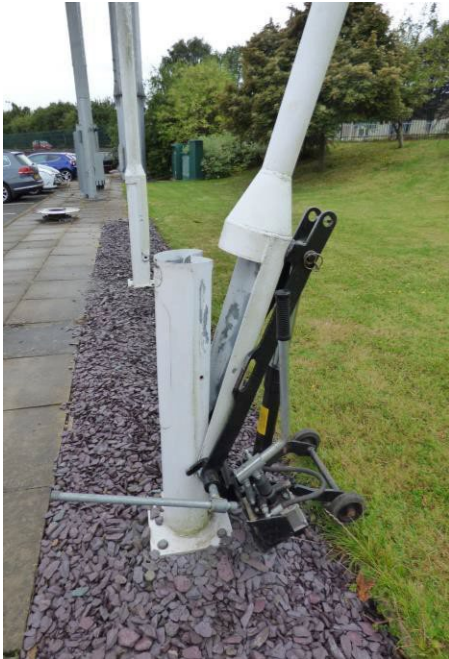
3. Open the control valve to start lowering
