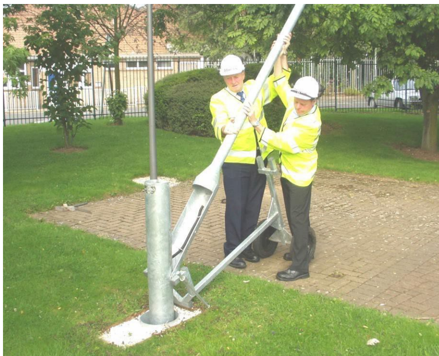
Figure 10-4 - Raising the column to a vertical position
